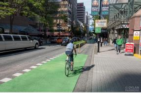
Green pavement, bicycle symbols, elephant's feet and bicycle signals at signalized intersection on a two-way
