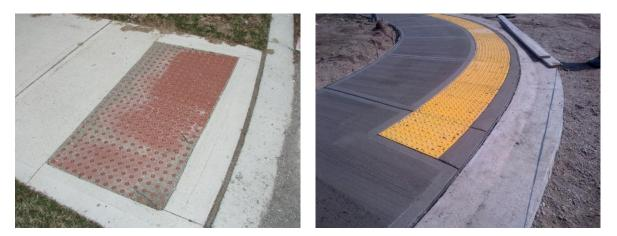
Example of cast iron tactile walking surface indicator, London ON and new installation Kitchener ON
