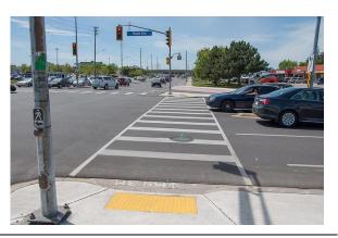
**Pedestrian pushbutton placement:** AODA Regulation 413/2 requires the accessible pedestrian signal push-button to be located within 1.5 m of the curb, a max. of 1.1 m above ground level and 3 m a part if there are two at the same corner). It must be in reach of the accessible sidewalk and near the curb ramp.
